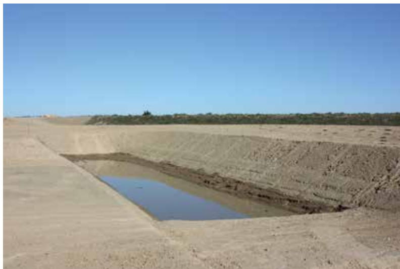
Figure 23: Vidourle jobsite: view of the F1 soil basin treated with 2% lime after 6 months (INRAE photo taken on 04-02-2016)
