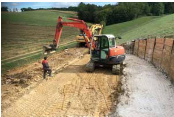
Structure with terraced benches (Photo: Lhoist)
