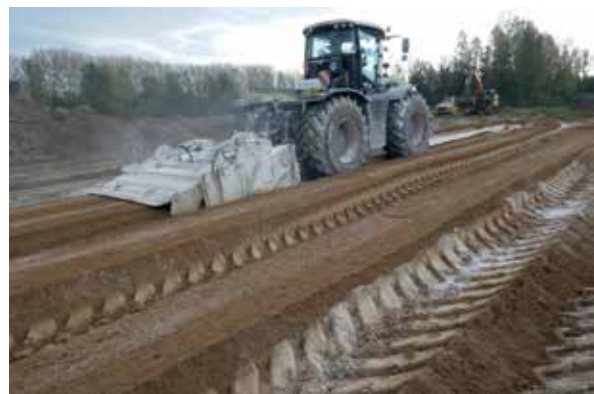
Tractor-mounted mixer (Vlassenbroek experimental jobsite – Photo: Lhoist)
