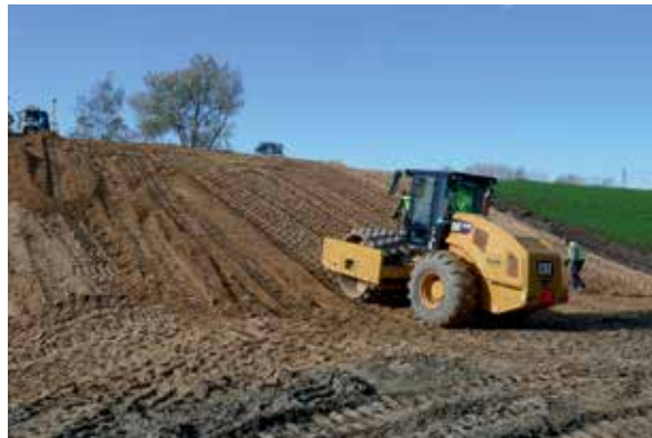
Figure 47: Compaction of a layer along a 3H:1V slope (Vlassenbroek experimental jobsite – Photo: Lhoist)
