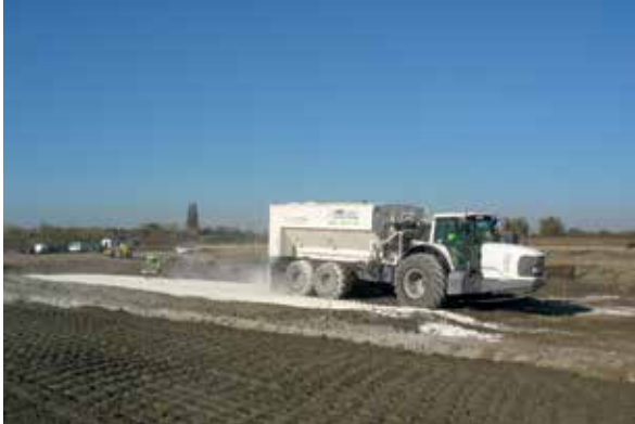
Lime spreading on the dedicated soil treatment platform with a volumetric dosing spreader and weight control (Salin de Giraud jobsite, November 2017 – Photo: Lhoist)
