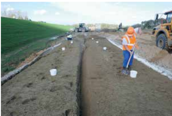
Taking samples for water content measurement on a field test (Photo: Lhoist)
