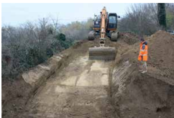
Earthworks of an existing structure (Photo: INRAE)
