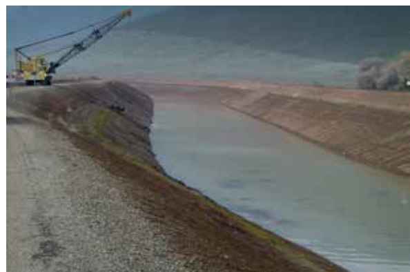
Surface cleaning after canal drainage (Lhoist photo)
