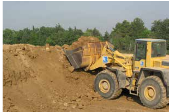
Loading for temporary storage to supply a treatment plant (Photo: DigueELITE)
