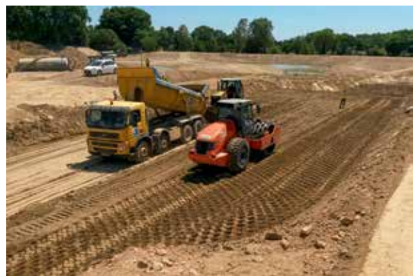
Simultaneous execution of implementation and compaction operations (Vidourle jobsite – Photo: DigueELITE)
