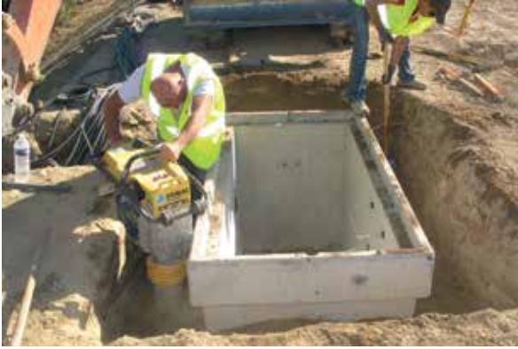
Compaction with a vibratory tamper around a manhole (Photo: DigueELITE)
