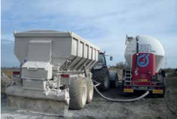
Visual check of spreader loading without dust emission (Photo: Lhoist)
