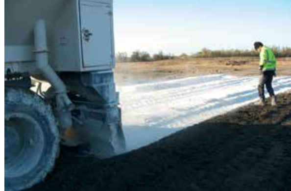
Visual check of lime spreading without dust emission (Photo: Lhoist)
