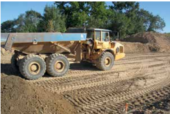
Movement of a dumper on F1 soil at the Vidourle jobsite (Photo: DigueELITE)
