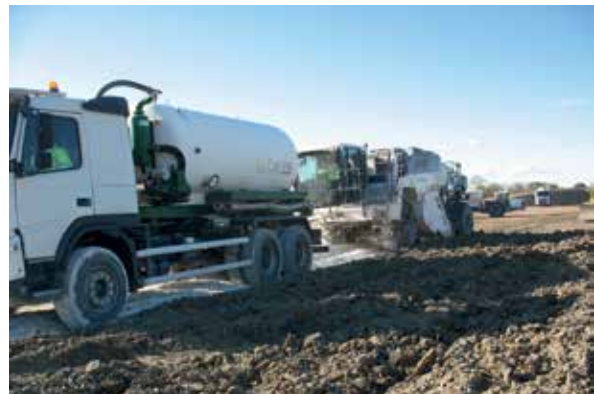
Combined watering and mixing machinery: the sprinkler is pushed by the self-propelled mixer, and water is incorporated directly into the mixer drum (Salin de Giraud jobsite November 2017 – Photo: Lhoist)
