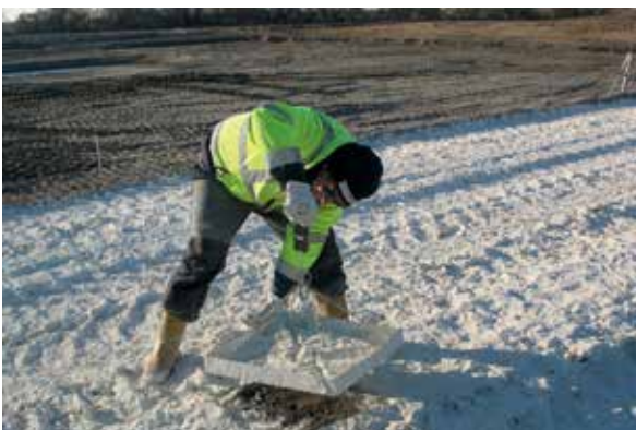
Control of spread lime surface mass by pan weighing (Photo: Lhoist)
