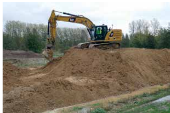
Homogenization of natural soil using an excavator on a temporary stockpile (Vlassenbroek experimental jobsite - Photo: Lhoist)
