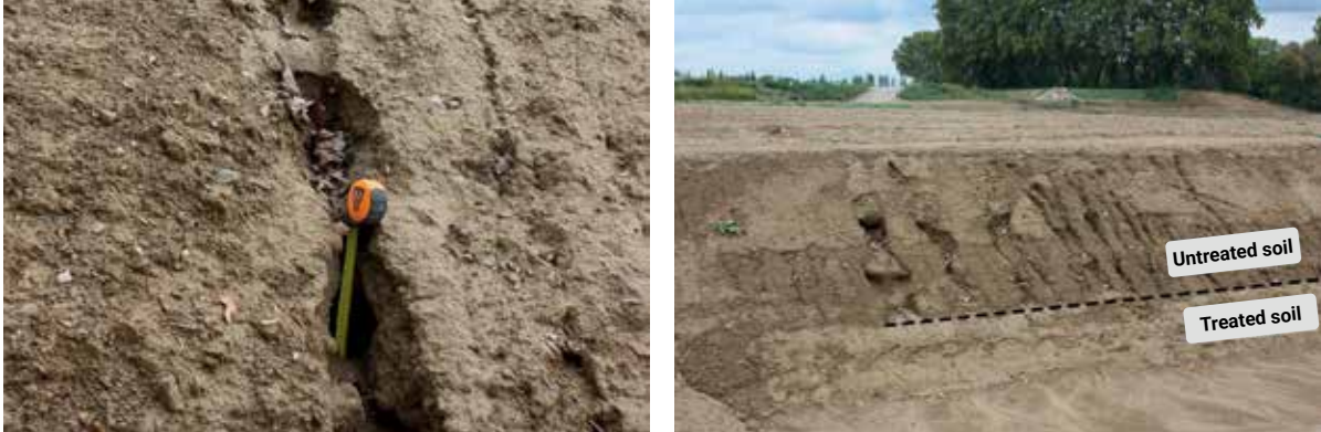
Erosion gully in the untreated soil on the left and behavioral contrast between lime-treated soil (smooth slope) and untreated soil (gullied slope) on the right (construction + 3 months) (DigueELITE photos)
