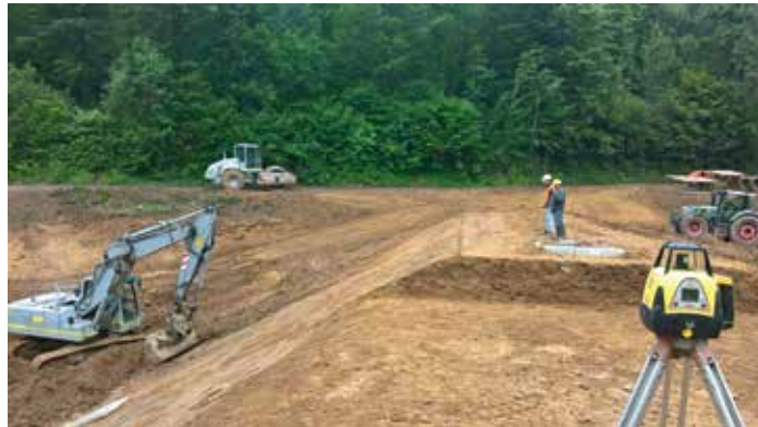
Figure 54: Trimming of slopes for a hillside retention structure (Photo: Entreprise Lhotellier)
