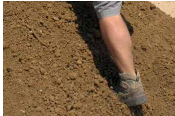
Detail of the grain size of F1 soil treated with 2% CaO at the treatment plant outlet (Vidourle DigueELITE project experimental jobsite)
