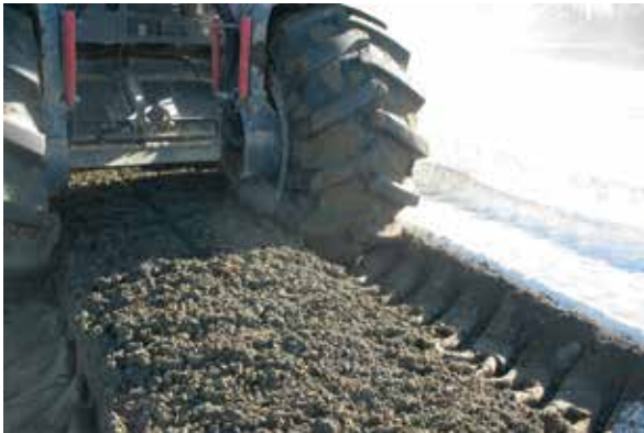
View of the grain size of F1 soil treated with 2% CaO after one mixer pass (Salin de Giraud jobsite November 2017 - Photo: Lhoist)
