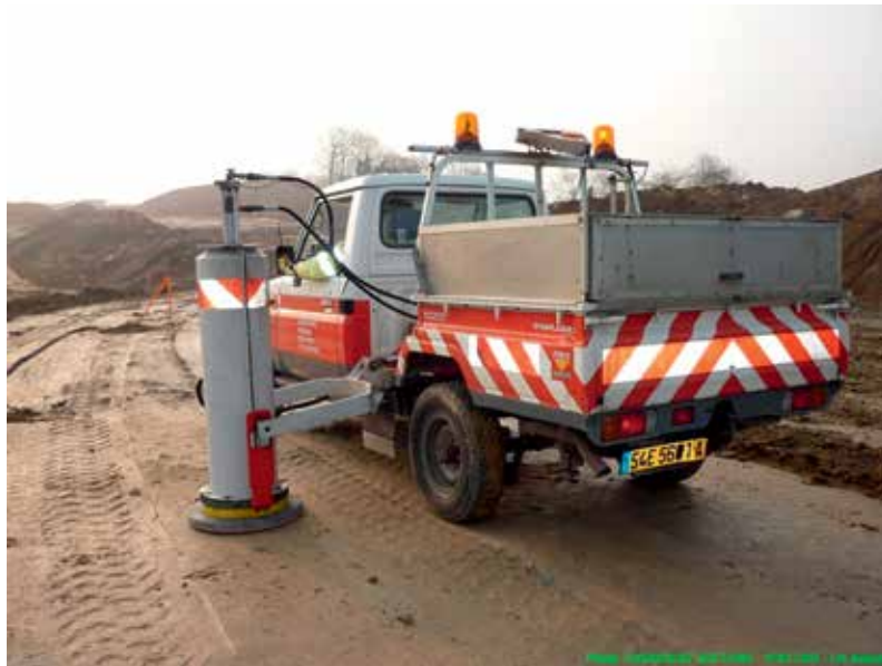
Figure 24: Bearing capacity measurement with dynamic plate load tests on a subgrade capping layer in F3 soil treated with 5% CaO (experimental worksite RD438 at Héricourt), (TerDOUEST project photo)
