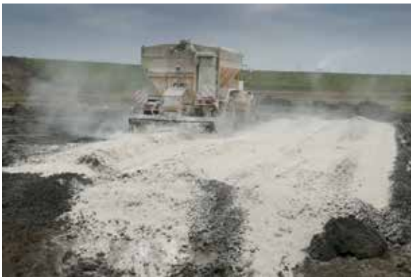
Lime spreading on a wet F2 soil with a volumetric dosing spreader (Photo: Lhoist)
