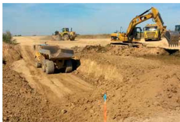
Earthworks for a F2 soil deposit (Photo: DigueELITE)
