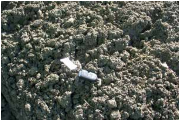
Detail of the grain size of F1 soil treated with 2% CaO after one mixer pass (Salin de Giraud jobsite November 2017 – Photo: Lhoist)
