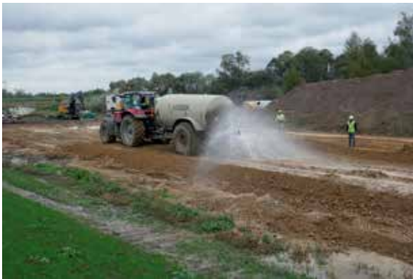
Watering of a natural soil platform with a "carp-tail" surface sprinkler (Vlassenbroek experimental jobsite - Photo: Lhoist)
