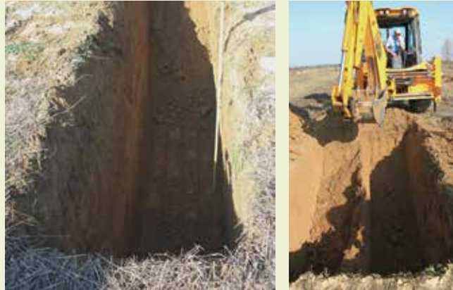
Exploratory surveys of the borrow area using an excavator
