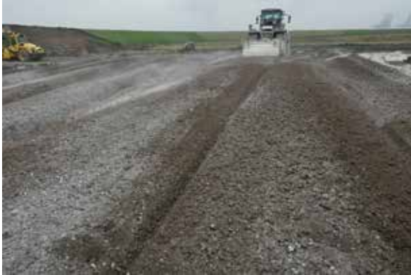
View of the grain size of F2 soil treated with 4% CaO after one mixer pass (Photo: Lhoist)
