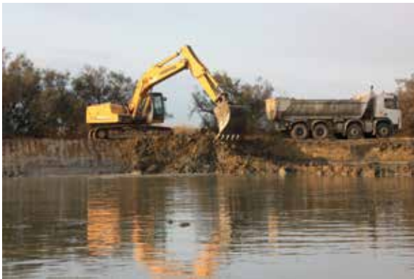
Excavation of a deposit with an excavator with homogenization (Salin de Giraud jobsite November 2017 - Photo: INRAE)
