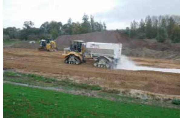
Lime spreading on a dedicated soil treatment platform with a tracked volumetric dosing spreader and weight control (Vlassenbroek experimental jobsite – Photo: Lhoist)
