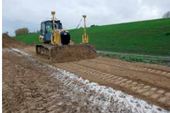
Spreading a layer of treated soil on a field test with a bulldozer equipped with an altimetric GPS system (Vlassenbroek experimental jobsite – Photo: Lhoist)
