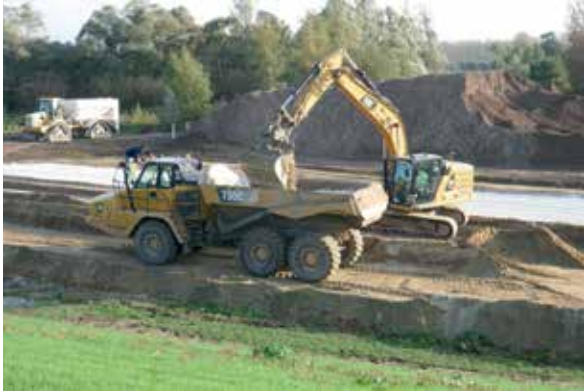
Recovery of treated soil with an excavator on a platform with GPS guidance; note that the string in the foreground has not been included as untreated (Vlassenbroek experimental jobsite – Photo: Lhoist)
