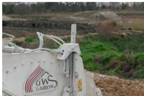
Inspection of the mixing depth indicator installed on the mixer (Photo: Lhoist)
