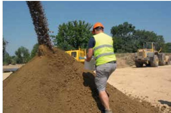
View of the grain size of F1 soil treated with 2% CaO at the treatment plant outlet (Vidourle DigueELITE project experimental jobsite)
