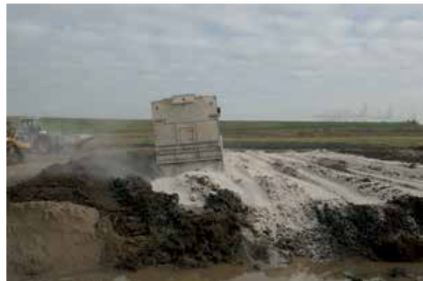
Lime spreading on a wet F2 soil with a tracked volumetric dosing spreader and weight control (Photo: Lhoist)
