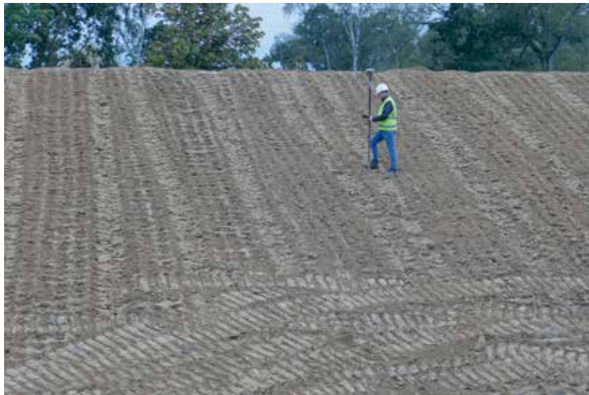
Figure 60: Final topographic survey by GPS (Vlassenbroek experimental jobsites – Photo: Lhoist)
