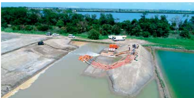
Figure 28 Experimental plots at Salin de Giraud – General view of the site (treated soil plot on the left and natural soil plot undergoing overflow tests on the right) (Photo: SYMADREM)
