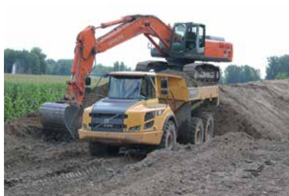
Soil recovery from a temporary stockpile (Photo: Lhoist)
