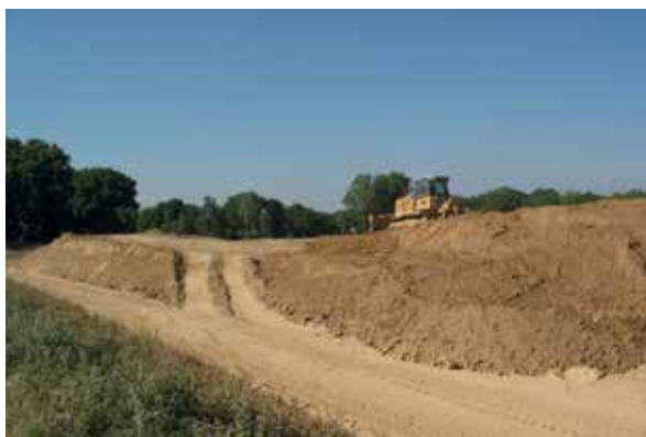
Creation of a temporary stockpile (Photo: DigueELITE)
