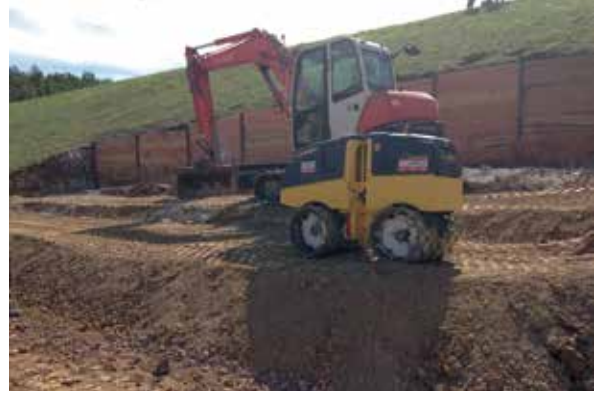
Small vibrating padfoot roller (Photo: Lhoist)
