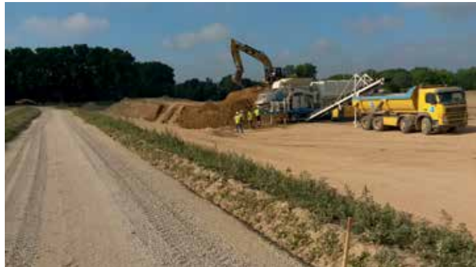
Temporary natural soil stockpile and mobile treatment plant (Vidourle jobsite July 2015) (Photo: DigueELITE)
