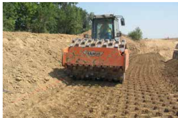
Compaction of an embankment without terraced benches, supported by the slope of an existing structure (Photo: DigueELITE)
