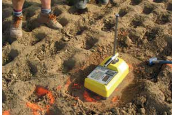
Figure 59: In-situ density measurement using a gamma densimeter (Photo: DigueELITE)
