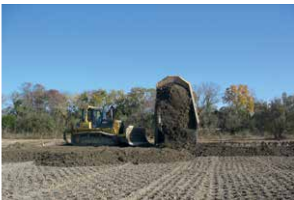
Supply of treated soil by dumper and spreading of a layer with a bulldozer (Salin de Giraud jobsite – Photo: Lhoist)
