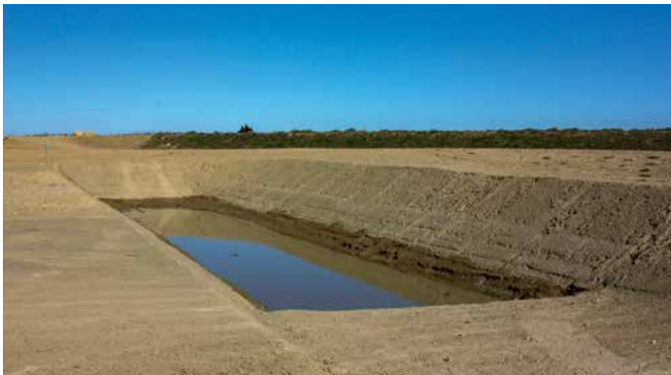
Water retention basin sealed by 2 compacted layers of lime-treated soil (DigueELITE photo)
