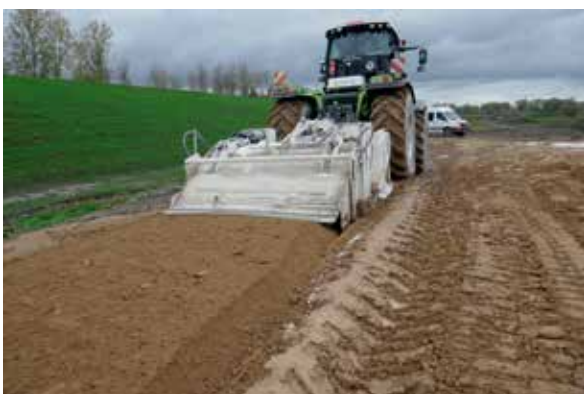
Mixing of natural soil after watering (Vlassenbroek experimental jobsite - Photo: Lhoist)
